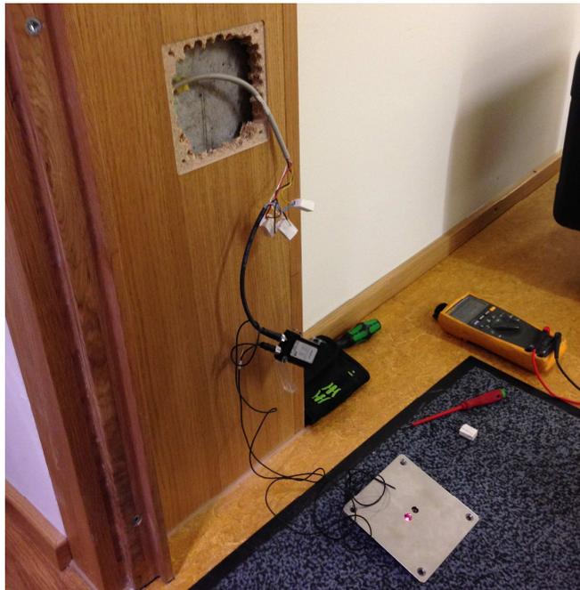
Fig. 3 Installation and setup of light barrier switch into doorframe
