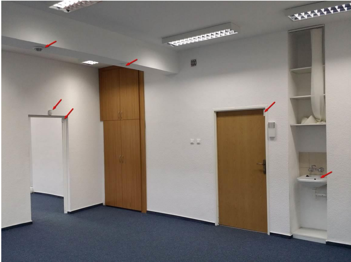
Fig. 1. PIA Integration Site – Room 1 – main entrance to the laboratory, wireless flood detector, wireless movement sensor, wire movement sensor, open-door detector.
