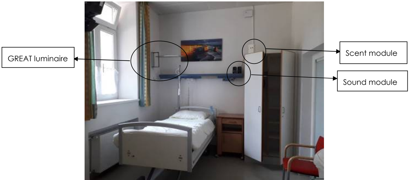
Figure 27: GREAT system implemented in a patient's room in the hospital in Hall (Austria)
