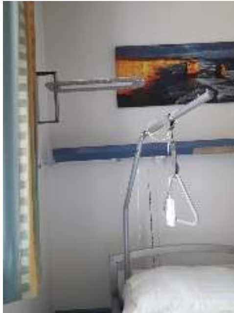
Figure 24: Wall-mounted GREAT luminaire in a patient's room in the hospital in Hall (Austria)
