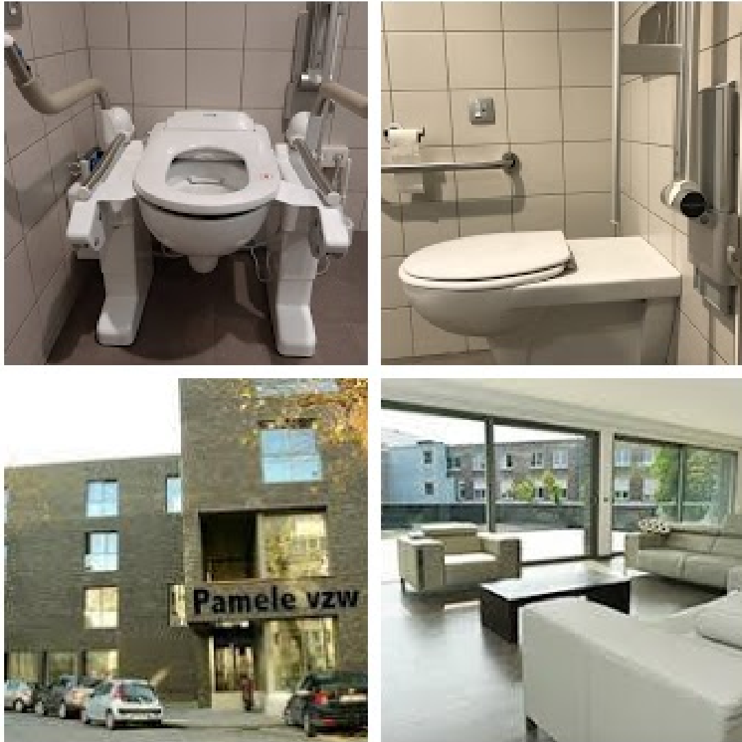
Figure 7: Test site 2 Pamele in Belgium: Toilet after installing the smart toilet: lift and shower WC. (above left) Toilet before (above right), building (bottom left) and living room (bottom right)
